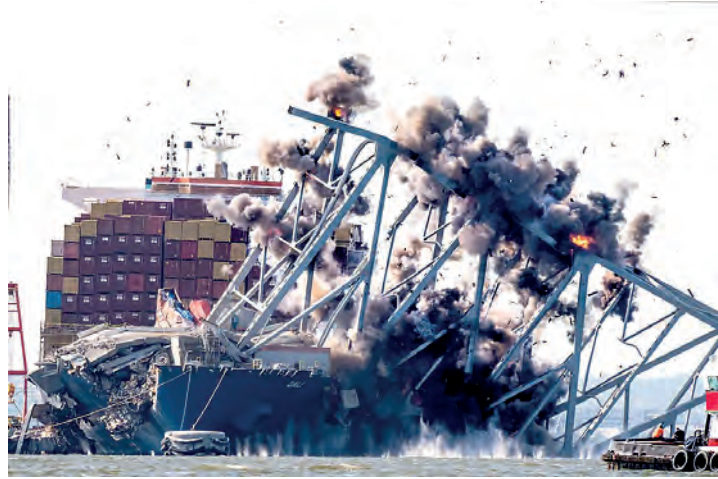
Baltimore, USA Crews conduct a controlled demolition of a section of the Francis Scott Key Bridge resting on the Dali container ship. The bridge collapsed on March 26 when the vessel lost power and collided into a support column, killing six construction workers. ◀
