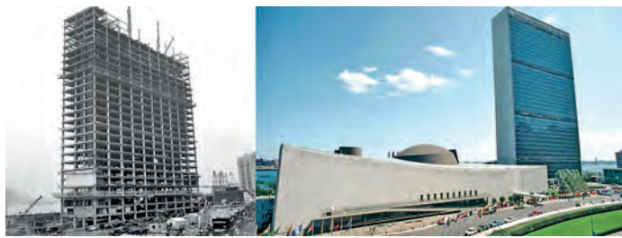
The UN Secretariat building (left) under construction in New York City in 1949, and the Secretariat and General Assembly buildings in 1990 (right). (UN Photo)
