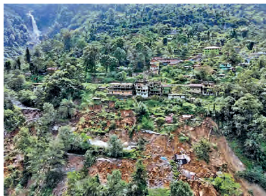
Naga-Namgor, India A drone view of damaged roads and houses that were washed away by flash floods in Sikkim.
