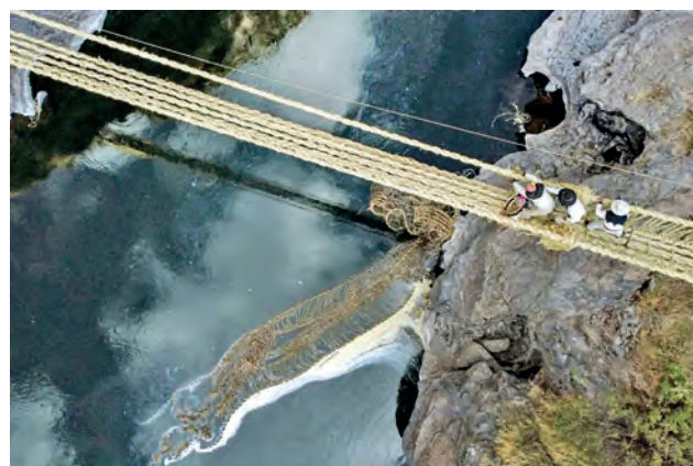
Huinchiri, Peru People from local communities participate in the annual rebuilding of the Q'eswachaka, the last remaining Inca rope bridge, as the old one drifts away in the Apurimac River.
