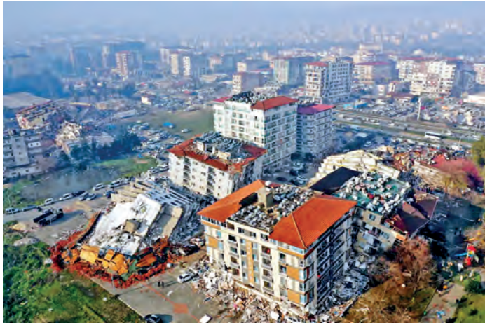
Hatay, Turkey An aerial view shows collapsed and damaged buildings after earthquakes struck near Turkey's border with Syria.
