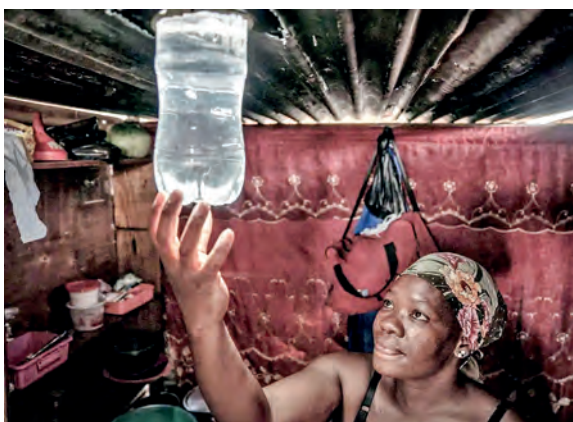
Olievenhoutbosch, South Africa Light beams out from a newly installed bottle globe inside a shack on an informal settlement in Centurion. The bottle globe provides daylight from a plastic bottle containing water and bleach that reflects sunlight. Scheduled blackouts, known as load-shedding, have burdened Africa's most industrialised economy for years.
