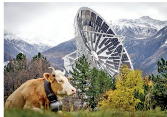
Leuk, Switzerland Old satellite dishes, which can be turned towards the sun, are lined with solar panels to generate winter power during a pioneering project in the Valais Alps.
