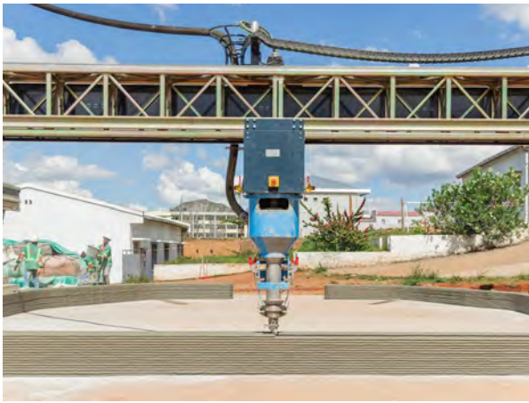
The 3D printer completed the walls of the school in 18 hours.
