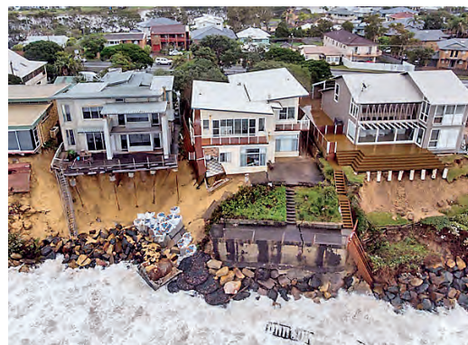
Terrigal beach, Australia Coastal erosion damages properties in New South Wales. A severe weather warning was issued for the coast from the southern border to Newcastle.
